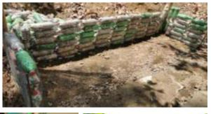
Walls of the Vermi house made of ecobricks
